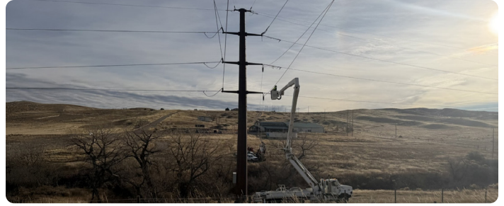
Waterton - Roxborough 115kv Transmission Line Rebuild
